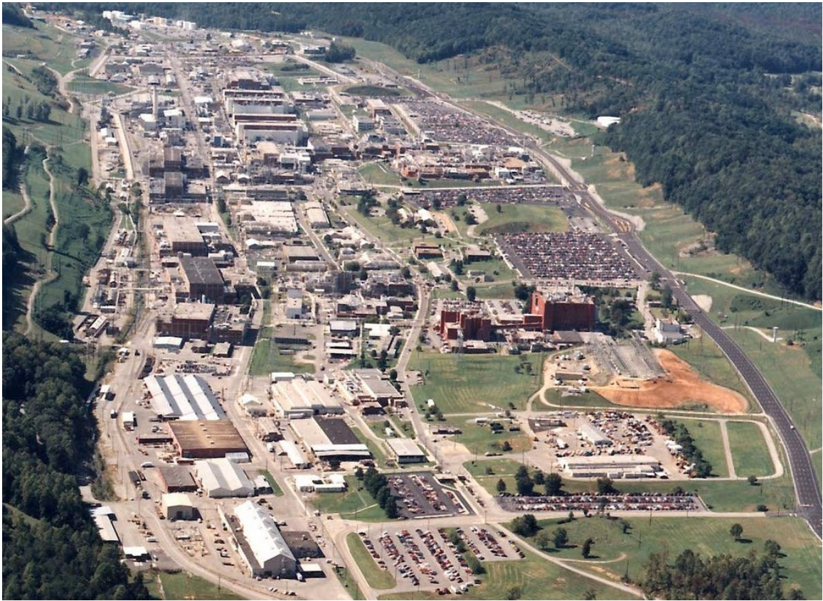
Figure 68. Y-12 Electromagnetic Plant
